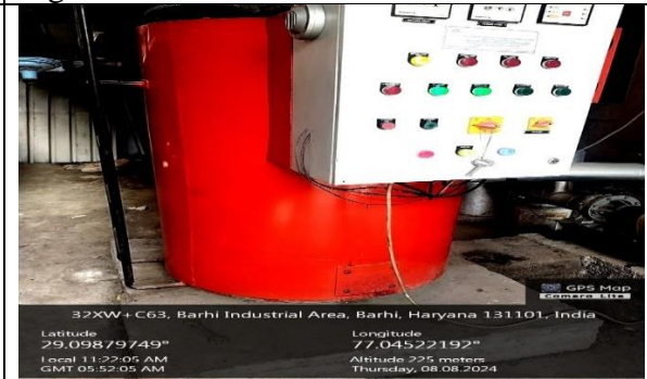
Fig.6: LPG Boiler
