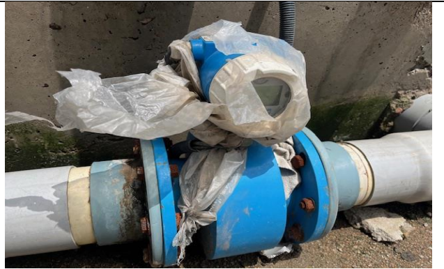
Fig.6: PETP outlet flow meter
