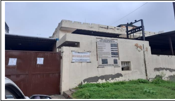
Entrance gate of the Unit
