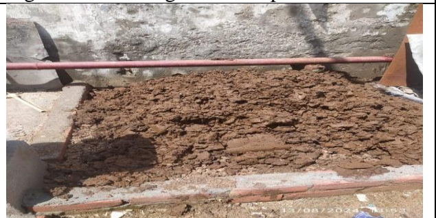
Fig.12: PETP unit (sand filter & carbon filter)
