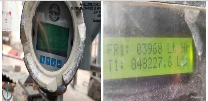
Fig.6: PETP inlet & outlet flow meter
