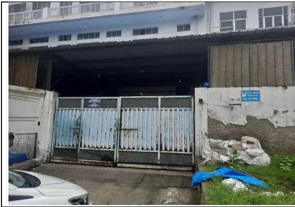
Entrance gate of the unit
