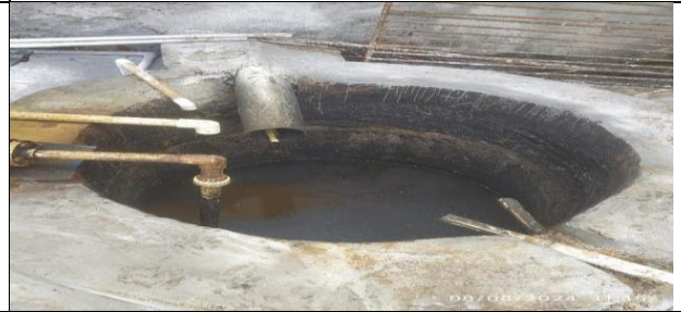
Photo 6: PETP Treatment Unit (empty & damaged tube settler)
