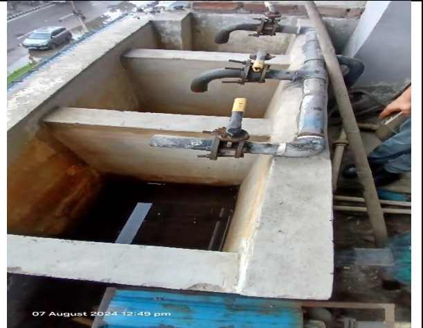
Photo 6: Sludge drying beds
