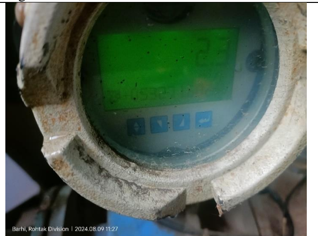
Fig.7: ETP outlet flow meter
