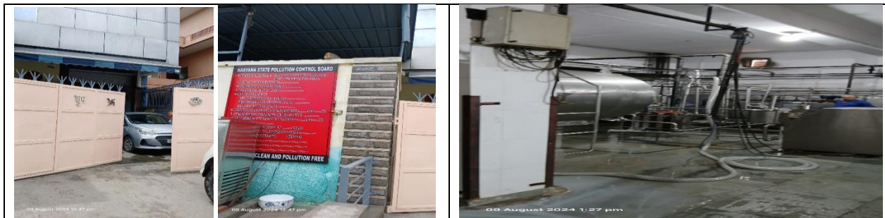
Photo 1: Entrance gate of the unit
