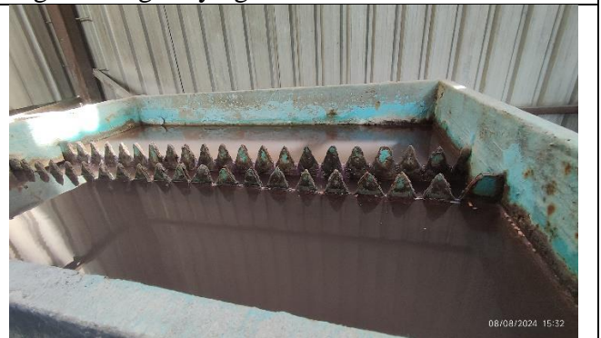
Fig.4: ETP Settling tank
