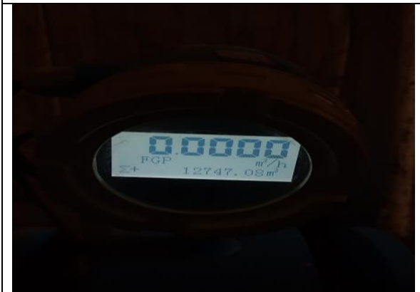
Flow meter installed at Borewell
