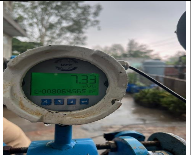
Fig.5: PETP outlet flow meter
