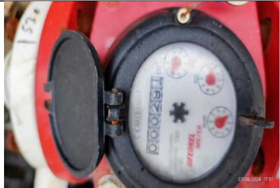
Fig: 10 Flow meter at the outlet ETP
