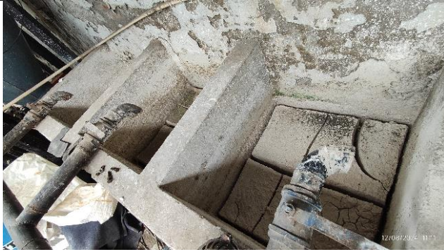
Fig.6: Sludge dry bed
