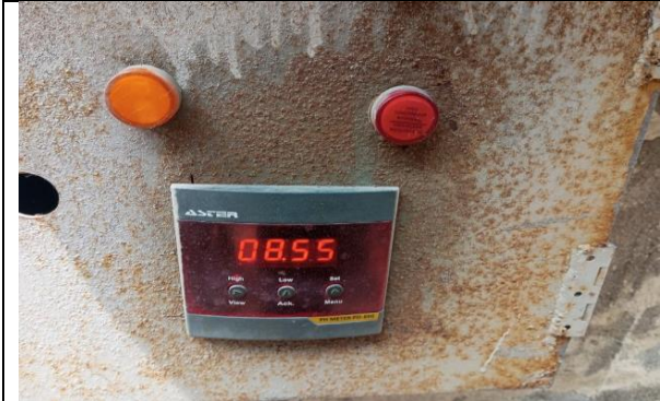
Fig.7: PETP inlet flow meter
