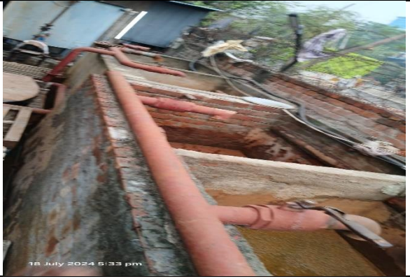
Photo 7: Sludge drying beds
