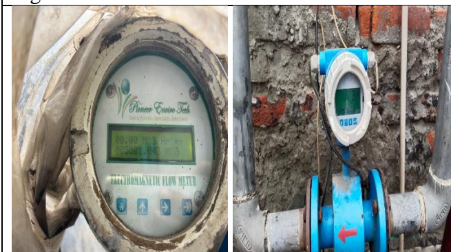
Fig.6: ETP inlet & outlet flow meter
