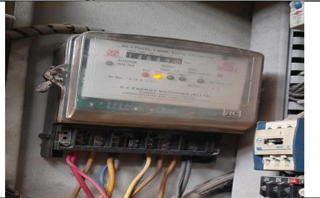
Energy meter installed at PETP
