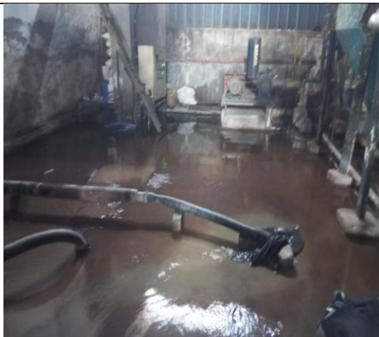
Fig.11: PETP area overflow from inlet collection tanks
