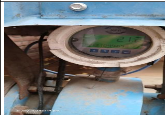
Photo 12: Flow meter on one Borewell
