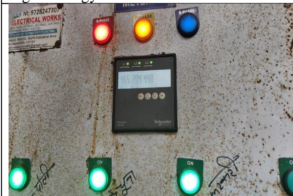
Fig.6: Energy meter of the ETP
