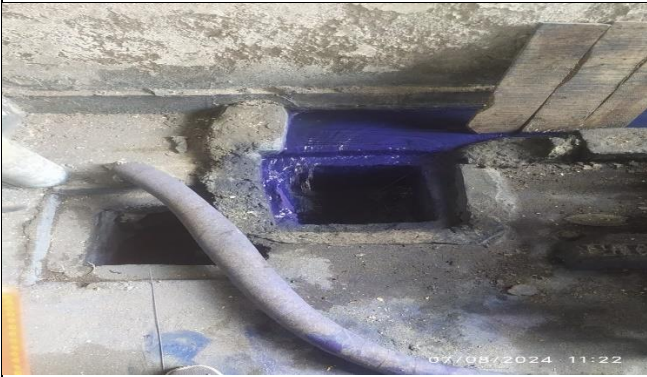
Photo 15: Loose pipe near Outlet chamber
