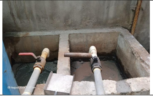
Photo 8: Sludge drying beds
