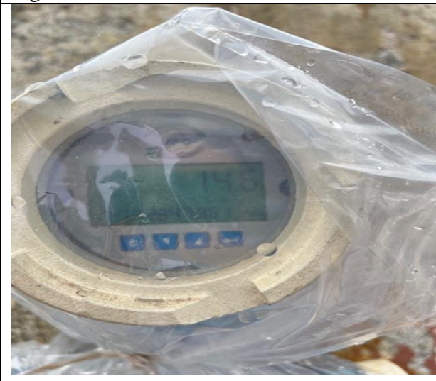
Fig.4: PETP inlet flow meter
