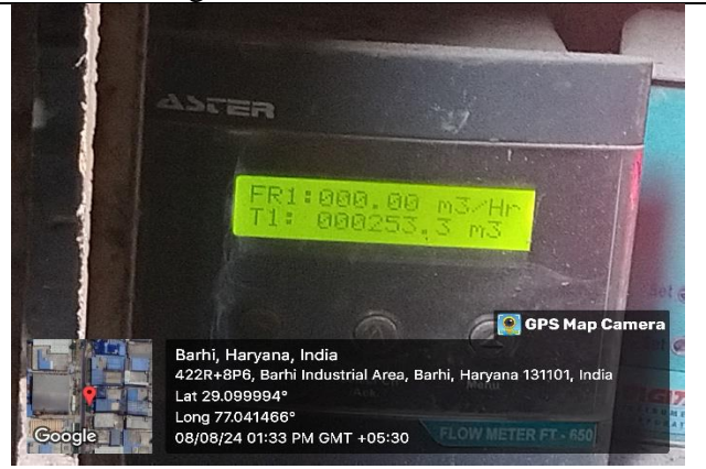
Fig.7: PETP outlet flow meter
