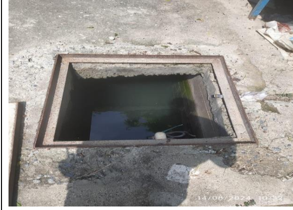
Fig.15: Rainwater harvesting pit in premises
