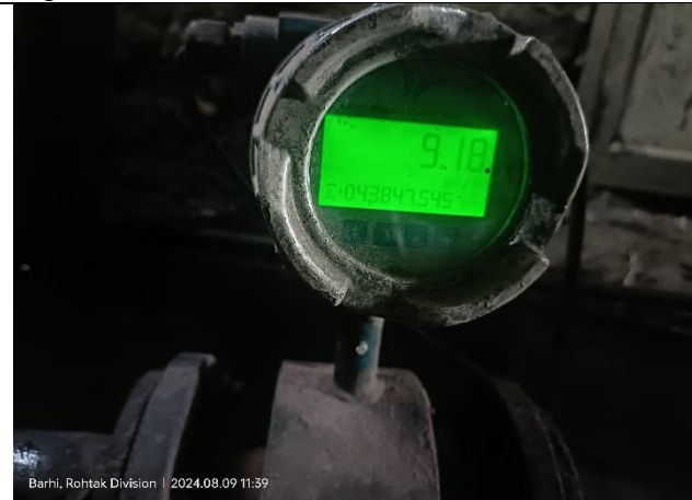
Fig.6: ETP inlet flow meter
