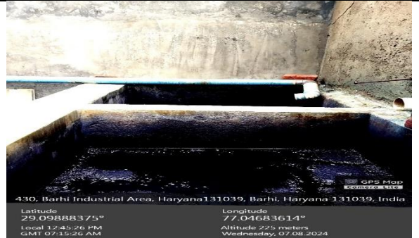
Fig.7: Sludge Drying Bed
