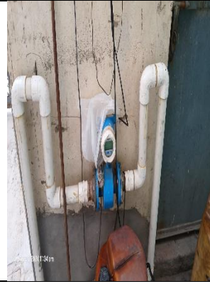
Photo 7: Tertiary treatment (Filtration) system & outlet flow meter
