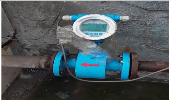
Fig.7: PETP outlet flow meter
