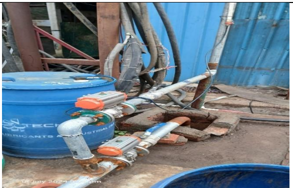
Photo 11: Installation of Treated effluent recycling system under progress
