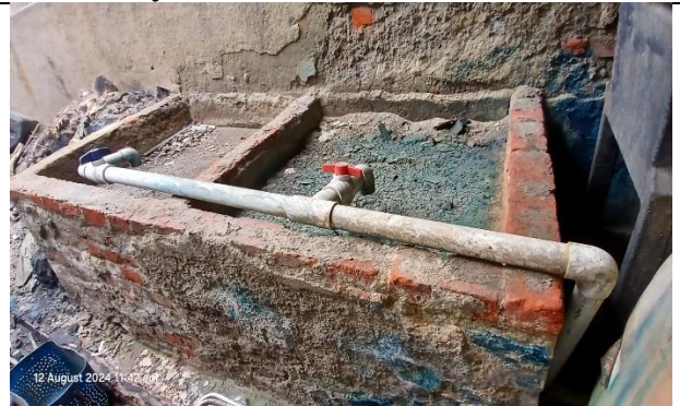
Photo 8: Sludge drying beds
