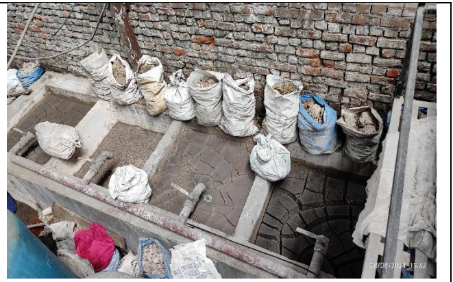
Fig.2: Sludge drying bed
