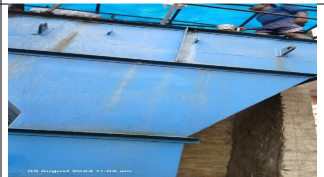
Photo 6: Chemical reaction tank & tube settler
