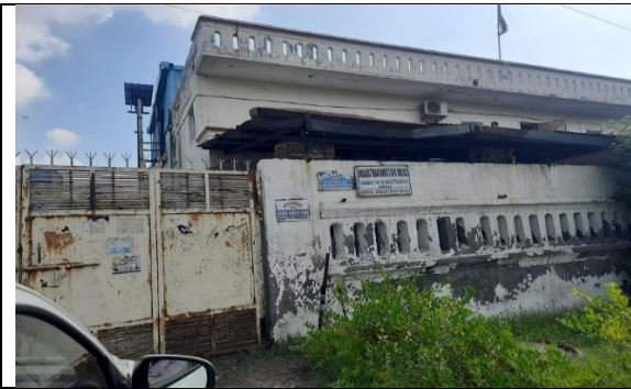
Entrance gate of the Unit
