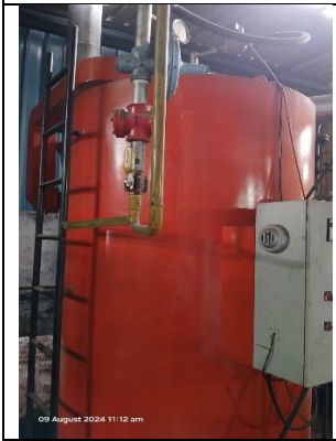
Photo 11: Thermopack & Briquettes as fuel
