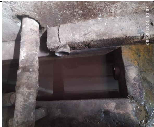
Direct outlet from process area to bypass channel
