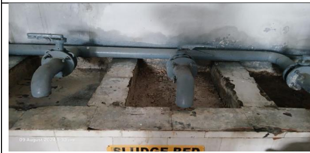
Photo 9: Sludge drying beds
