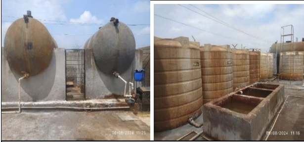
Photo 5: PETP Treatment Unit (Chemical dosing & mixing tank)
