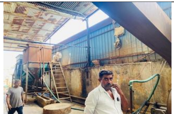
Fig.4: ETP set up
