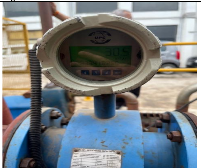
Fig.6: PETP outlet flow meter
