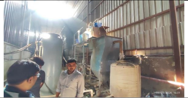
Fig.4: ETP set up
