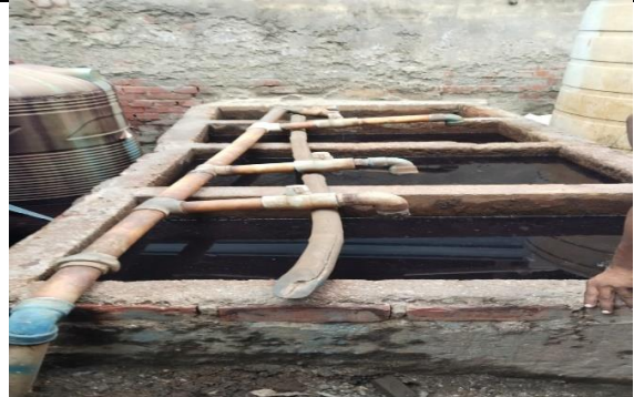
Fig.9: Sludge Drying Bed
