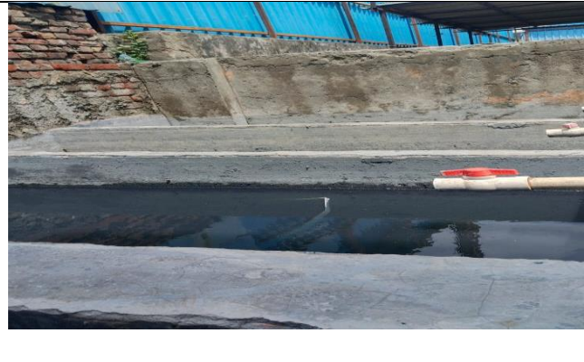
Fig.7: Sludge Drying Bed
