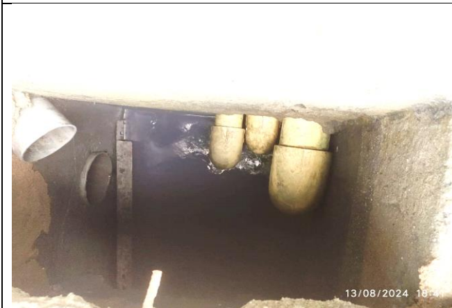
Fig.13: PETP outlet (with multiple pipelines)
