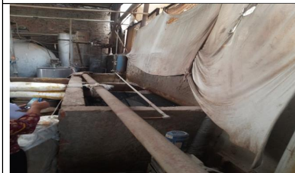
Sludge drying beds
