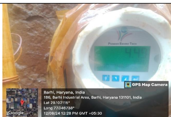
Fig.4: PETP outlet flow meter
