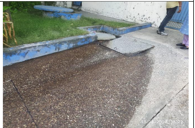
Fig.14: overflow at PETP outlet connection into HSIIDC sewer line.
