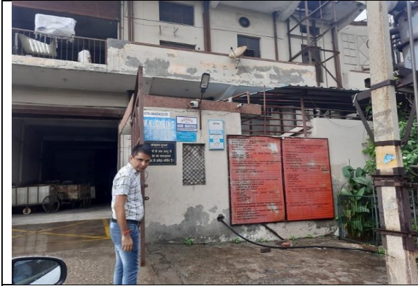
Entrance gate of the unit
