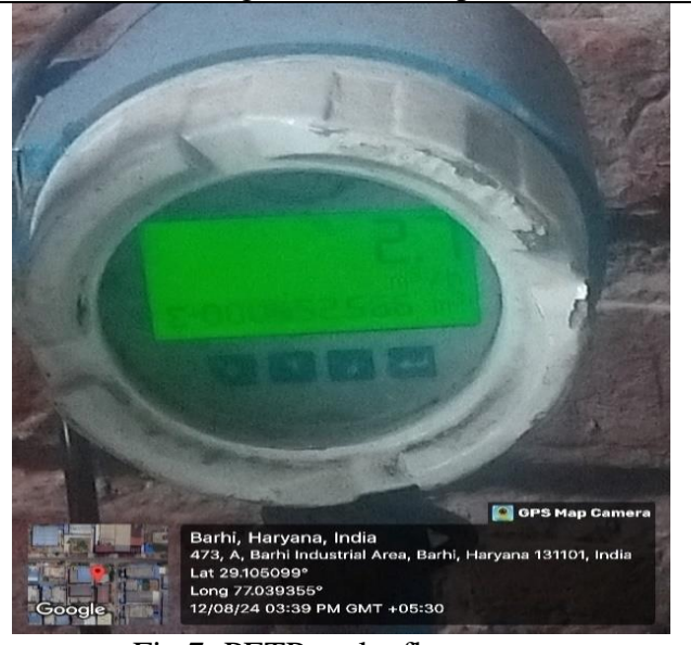
Fig.7: PETP outlet flow meter
