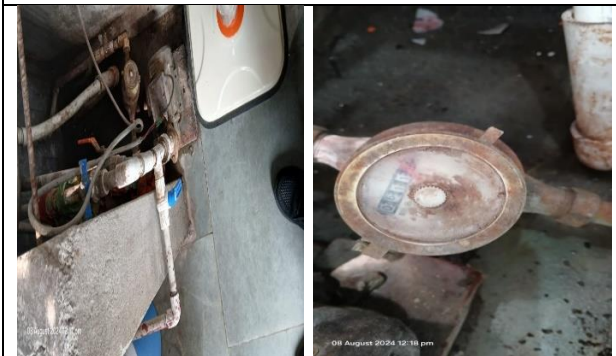
Photo 5: HSIIDC water supply with flow meter
