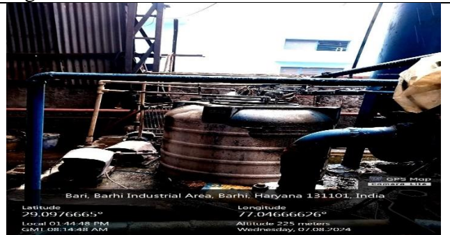
Fig.6: Dual Media Filter
