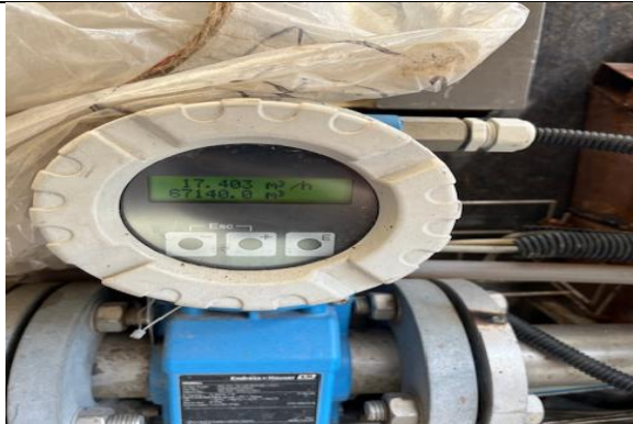
Fig.5: PETP inlet flow meter
