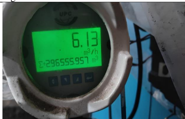
Fig.7: ETP outlet flow meter
