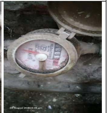
Photo 4: HSIIDC water supply line meter
