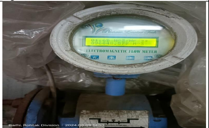
Fig.6: Flow meter at ETP outlet
