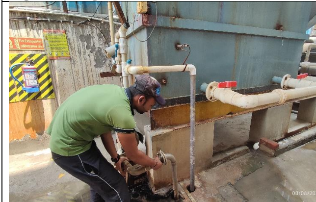
Fig.5: Inlet pump under maintenance
