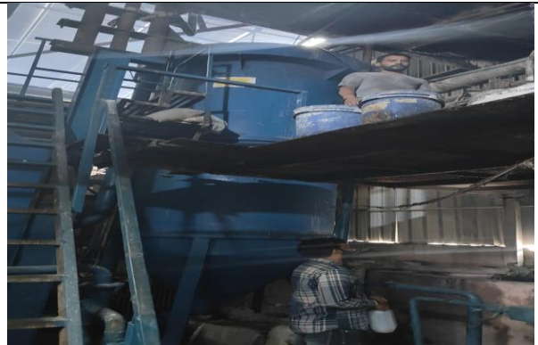
Fig.6: Flow meter at borewell
