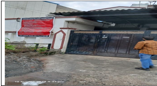
Photo 1: Entrance gate of the unit
