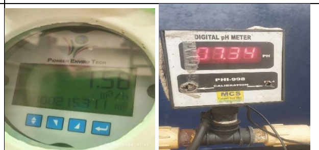
Photo 10: PETP outlet Flowmeter & pH meter at outlet
