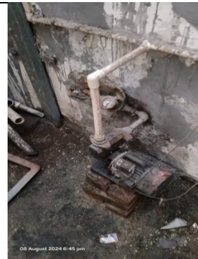
Photo 4: HSIIDC water supply line meter
