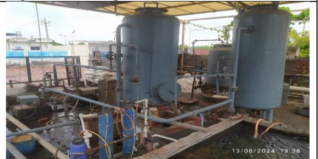
Fig.10: Softener plant for Boiler
