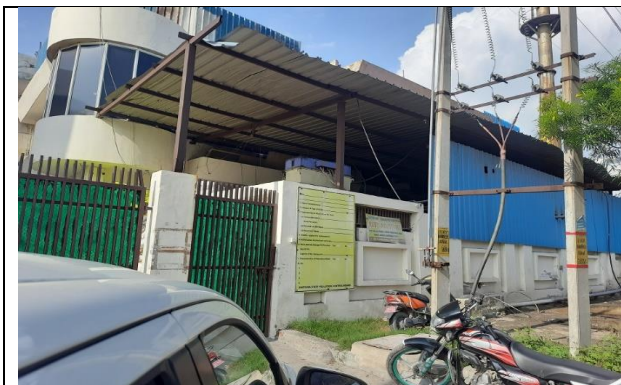
Entrance gate of the unit
