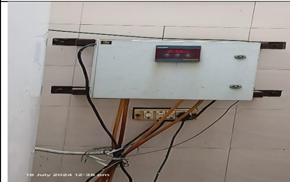
Photo 7: pH sensor at PETP outlet
