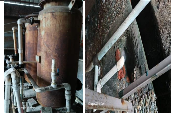
Photo 7: PETP Tertiary filtration units & outlet
