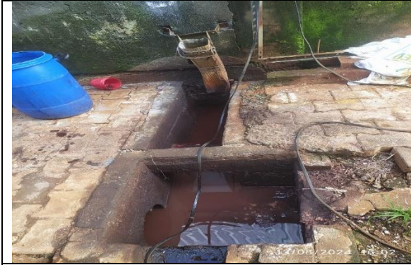
Fig.7: PETP inlet flow meter
