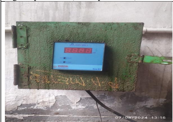
Fig.11: pH meter (Non-operational)
