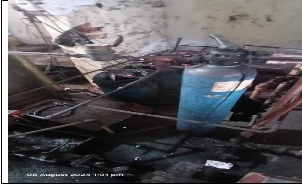
Photo 5: Tertiary treatment (Filtration) system
