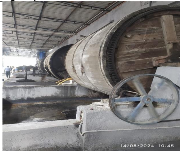
Fig.3: Drums adjacent to stormwater collection channel having only 4 inch height wall
